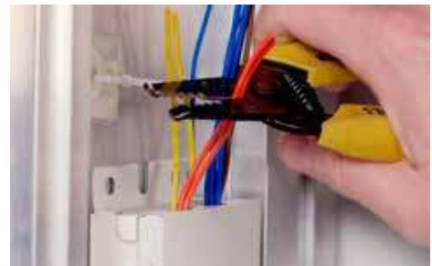
**2** Cut input and output wires on ballast.
