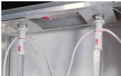
**3** Mount tubes in existing sockets or use spring-loaded brackets (available as accessories) if sockets are unable to hold lamp.
