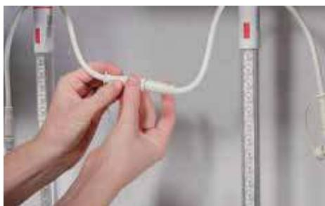
**6** Connect lamps together with waterproof cables.
